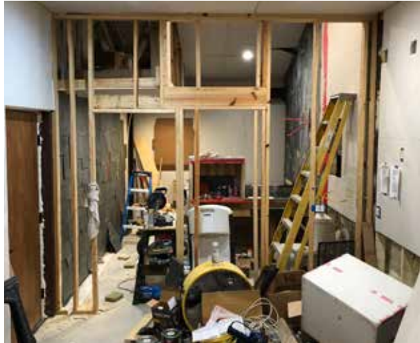
FINISHING WORK // APRIL 2019 - MAY 2020
