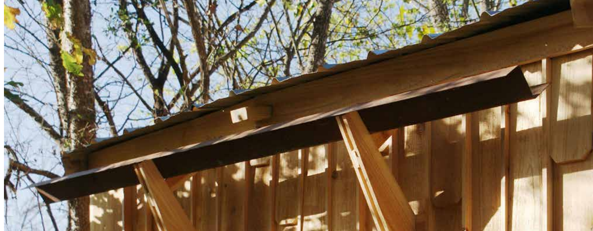
GUTTER DETAIL // SIMILAR TO THE DETAIL ON THE TRUSSES UNDER THE OVERHANG, THE GUTTER HIS HELD UP BY TWO ARMS MADE TO FIT A Z-BEAM. THIS BEAM WAS LEFT OVER FROM THE ARC'S CONSTRUCTION
